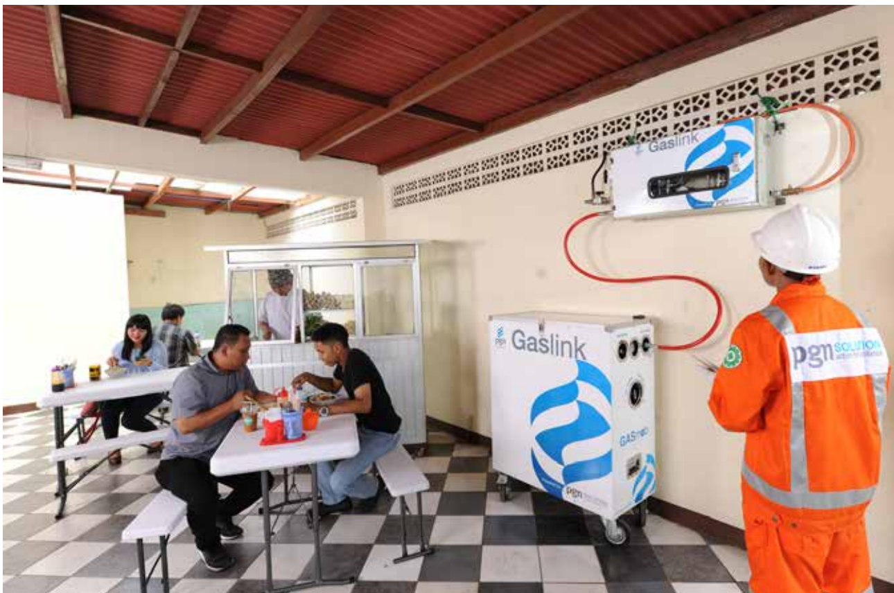
CNG Cradle (Gaslink), created by the PGASSOL Subsidiary for the support of the natural gas business in the commercial sector, especially for customers who have not crossed the gas pipeline. In addition to commas, PGASSOL also performs maintenance and operation of CNG Cradle.
