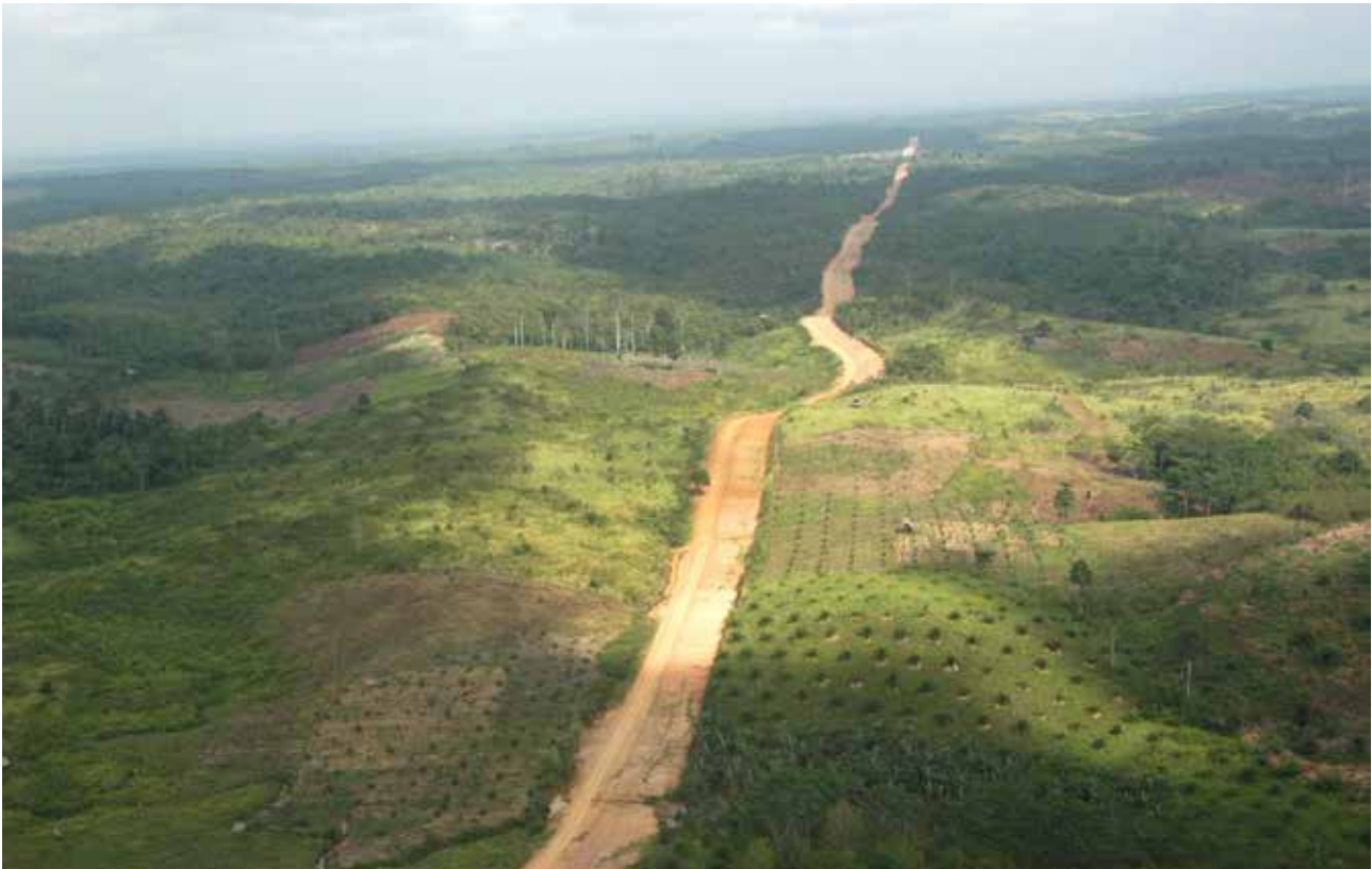
Gas transmission pipeline run by the TGI Subsidiary is located in a sterile location of residential and other objects. TGI manages and operates the pipeline with high security standards so that gas distribution from Sumatra Island to Java and Riau Islands can be done safely and stable.
