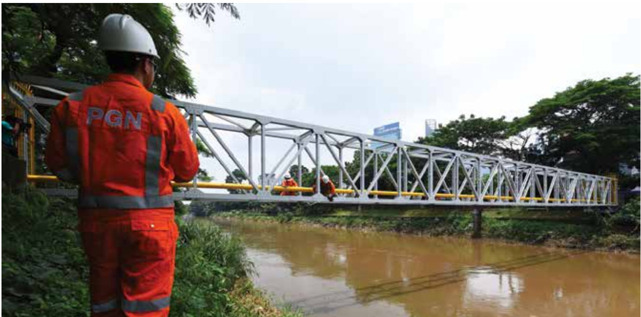
Natural gas distribution infrastructure operation, supervision, and maintenance was conducted in a regular routine with high security standard. PGN assigned a Subsidiary Entity, PGASSOL to manage the activity in all over Indonesia.
