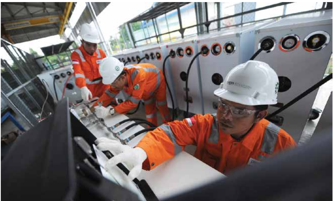
The subsidiary entity, PGASSOL, produced high quality CNG Cradle to support business development in providing commercial sectors that are missed from PGN's gas pipes. The business was maintained GEI, as a form of One PGN synergy.
