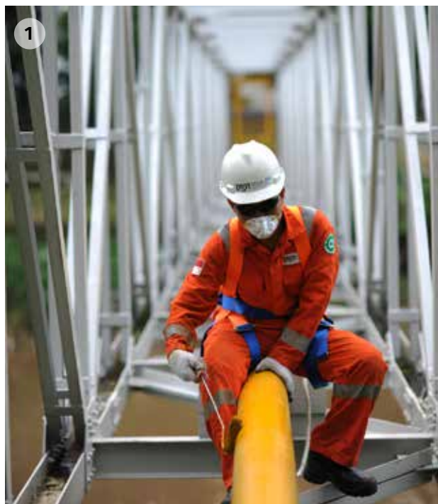
1. PGASSOL carries out maintenance and inspection of PGN’s gas pipelines with high security standards throughout Indonesia. 2. PGASSOL becomes an agent and distributor for a variety of quality gas equipment.
